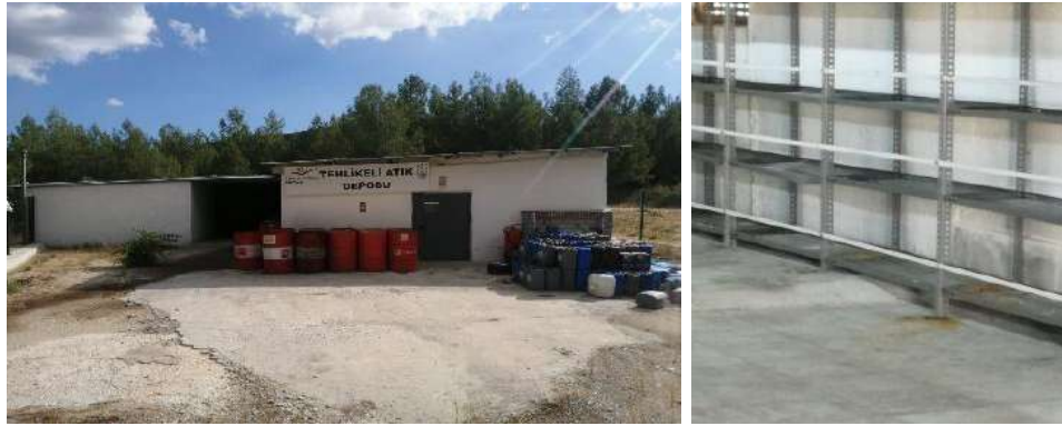
Figure 12: Hazardous Waste Warehouse
